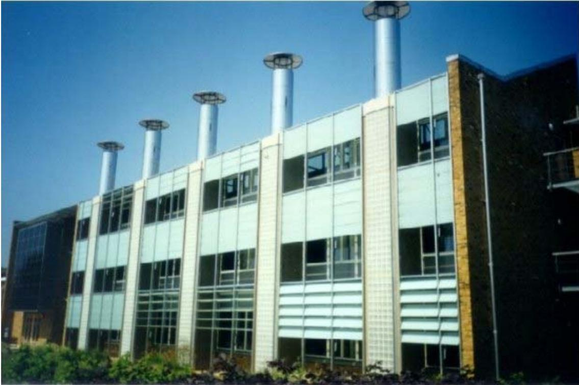
Figure 2. Modern office building with a blend of HVAC systems and classical features of natural ventilation. The BRE office building in Garston, UK uses among other features five wind towers to enhance natural ventilation.
